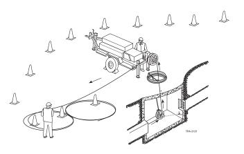
**4.11.** After the pulling eye is connected to the next section of the pull-line, feed the cable by hand back into the manhole and pull it to its next destination. The cable may be pulled directly from a figure-eight by a winch, provided the capstan or sheave used at the entry manhole ensures sufficient bend radius. Hand tending of cable paying off from figure-eights is normally required.
